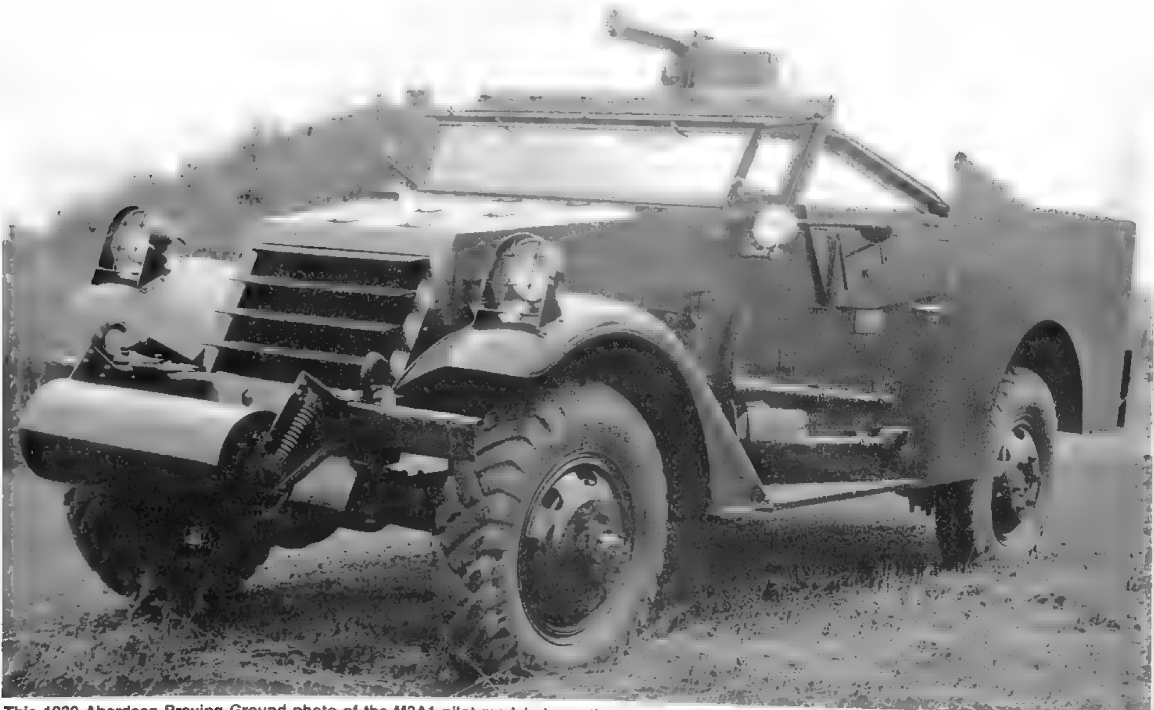
This 1939 Aberdeen Proving Ground photo of the M3A1 pilot model shows the protruding "greenhouse" windshield used on the earliest production vehicles. Also visible are the crossed swords of the cavalry on plaques mounted to the driver's door. Just ahead of the door is the chrome-plated spotlight. Both the latter details are repeated on the passenger's side of the vehicle. (National Archives and Records Administration photo)
